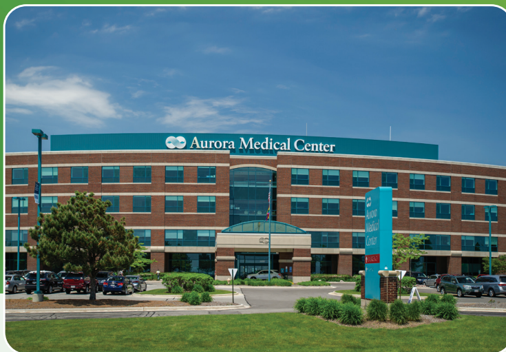
Aurora Medical Center – Manitowoc County, Two Rivers, Wis.
