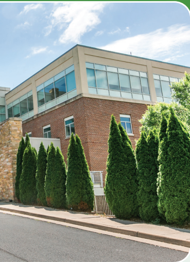
Carilion Rockbridge Community Hospital, Lexington, Va.
