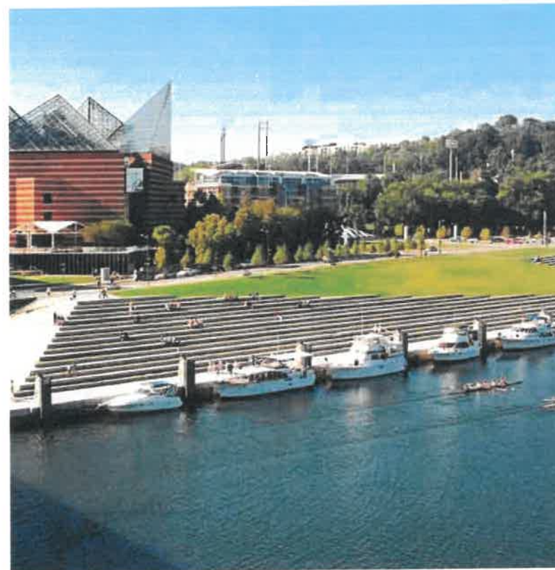
Example of transient dockage at seawall.
