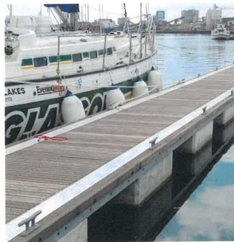
Example of floating side-tie dockage.
