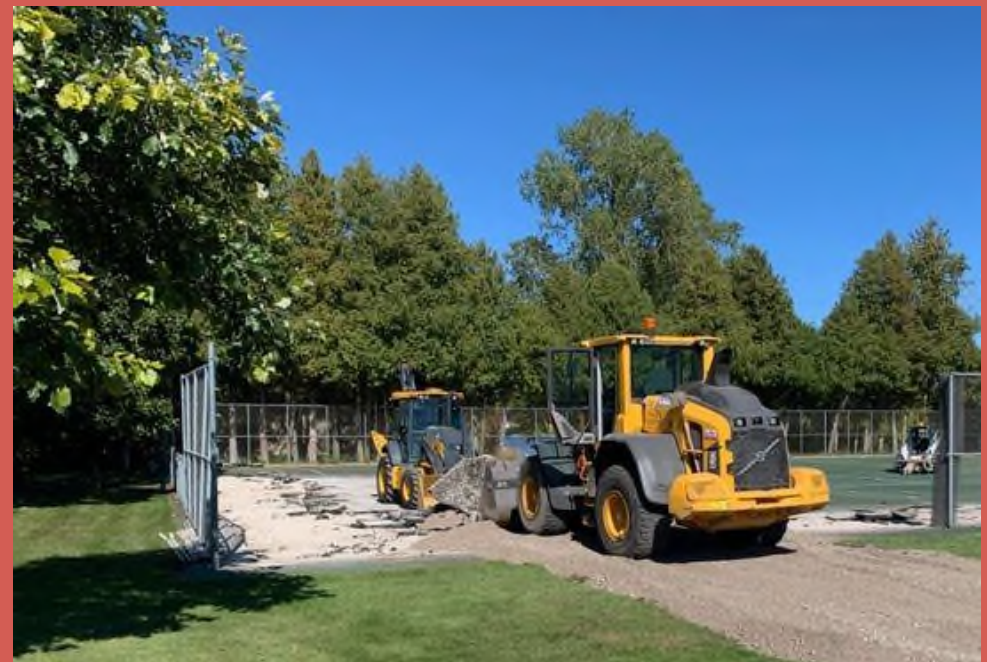
Pavement Removal by City Public Works Crews
