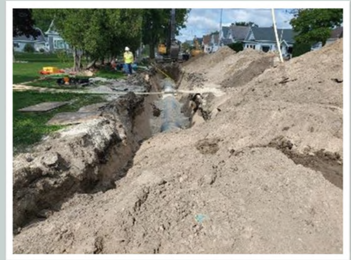
Storm Sewer Installation on 17 th Street
