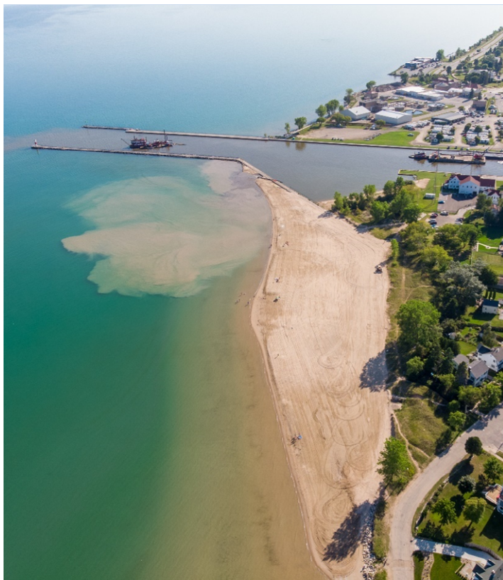
U.S. Army Corps of Engineers Dredging Summer 2020 ( photo courtesy MJH Photography )
