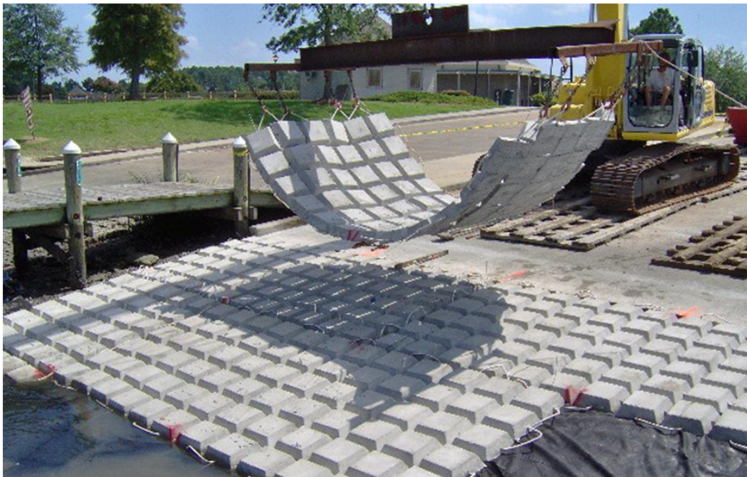
Figure 5: Example concrete mattress ramp
